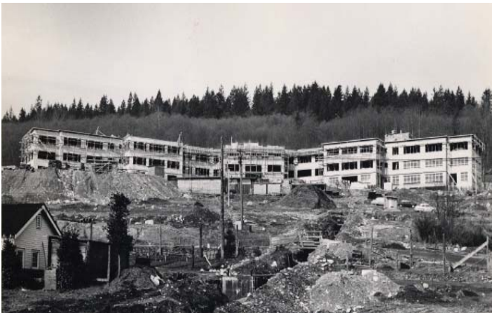
North Lawn under construction, March 1954
