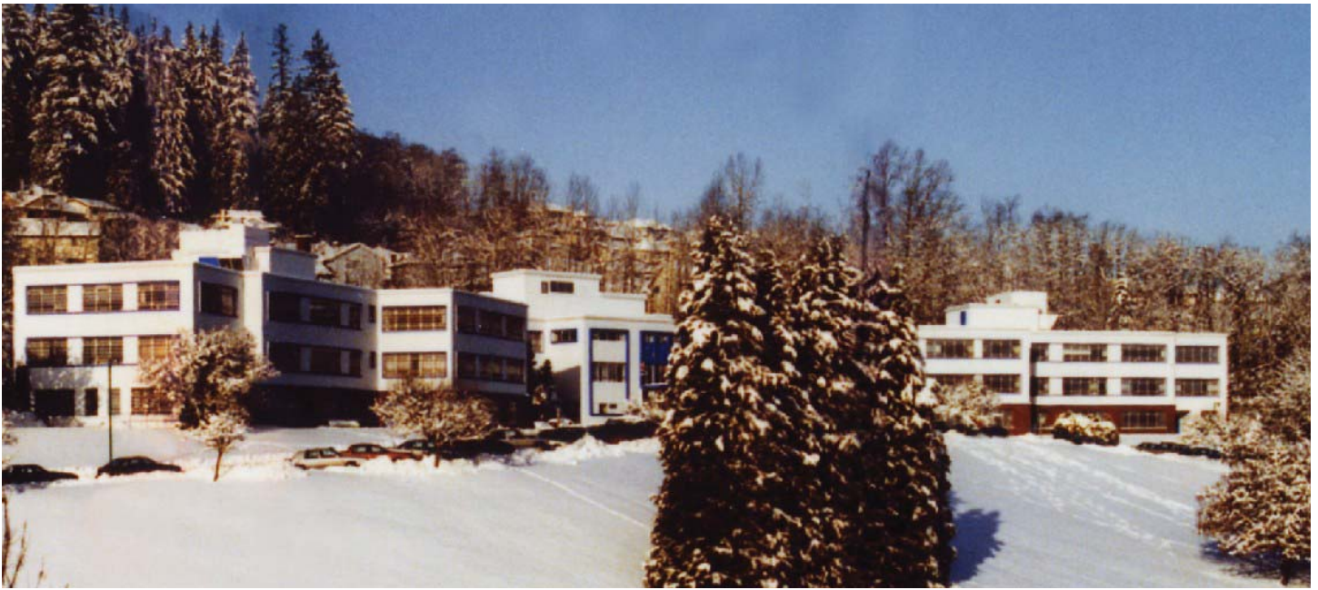
North Lawn building and grounds, winter 1989.
